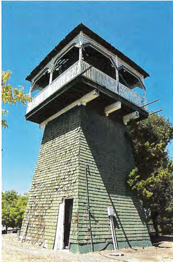
Figure 9. Oblique view of southeast (left) and northeast (right) facades, looking west.
