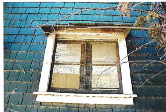
Figure 12. Window on northwest facade.
