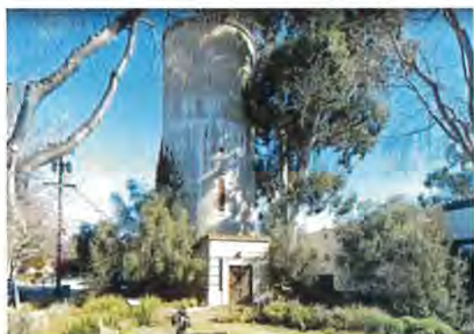
Figure 24. Fred Eyerly Water Tank/Tower Well at 10 Alma Street, Palo Alto. Source: PaloAlto.gov
