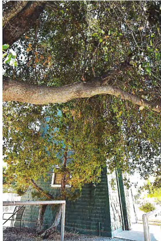
Figure 10. Northwest facade, looking southeast.
