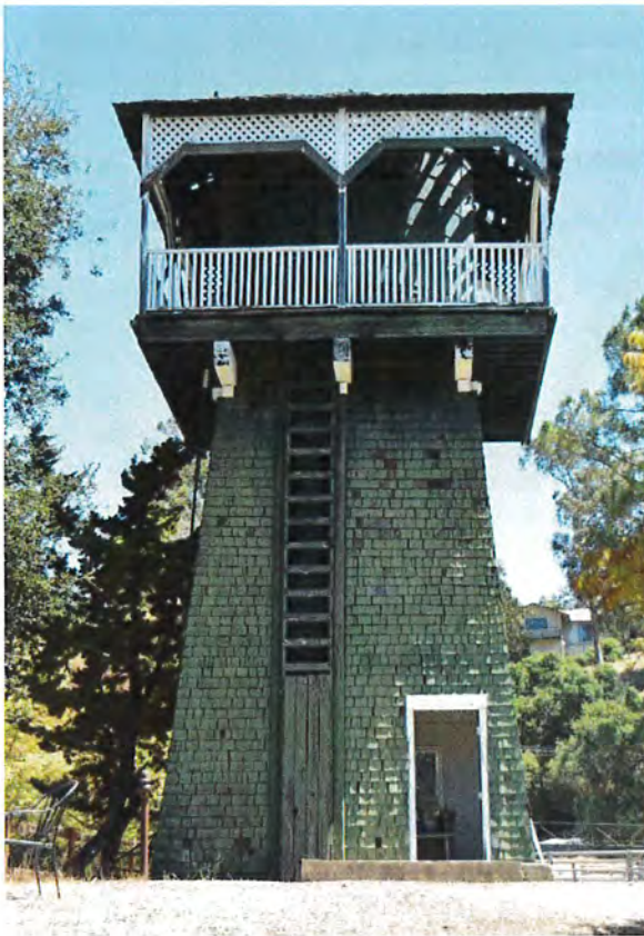
Figure 6. Southwest facade, looking northeast.
